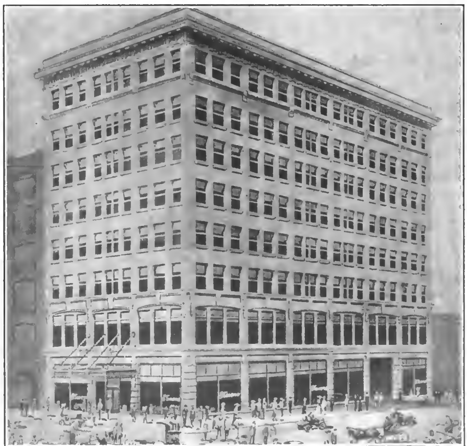
Building of the Pence Automobile Co., Stearns-Knight distributors in Minneapolis
